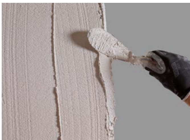
Render the surface areas, including the log store, but don't render the top of the log store areas (as granite will be placed there).
