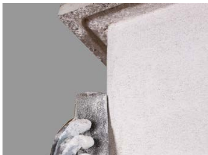
Smooth the render after completion.
