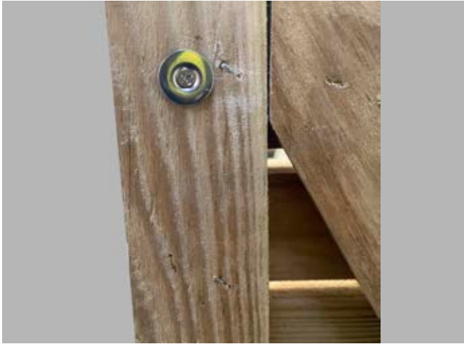
Attach the metal ring to the door.
