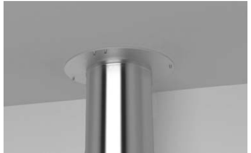
2-piece fire stop plate attached securely to joists.
