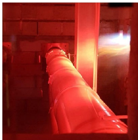
Stålskorstein under testing.
